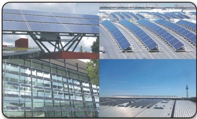
Solar power plant installations in Germany-aggregated to 36 GW.
